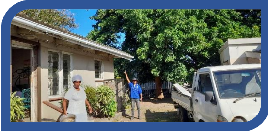
Gutters were replaced at Melville Hospice in KZN.
